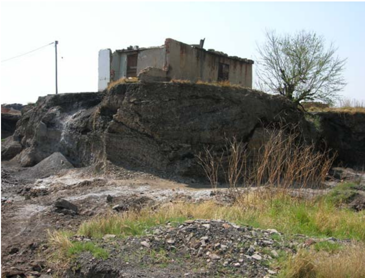
Figure 12: Blaaubosch – unstable house on edge of mine wall
